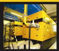
Combined or conjugated heat and power production (CHP – Combined Heat and Power) is when you produce electric power by means of burning fuel and you also utilise the heat and fume produced by the gas engine.
